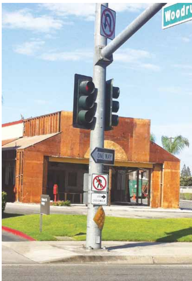
The El Pollo Loco at Firestone Boulevard and Woodruff Avenue is expected to stay open as it undergoes extensive remodeling, city officials said this week. The restaurant was closed earlier this week as workers stripped the building and gutted its interior.
