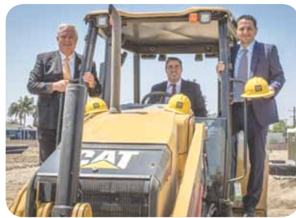
KB Homes broke ground on 117 townhomes that will replace the long-closed Gallatin Medical Center on Paramount Boulevard.
