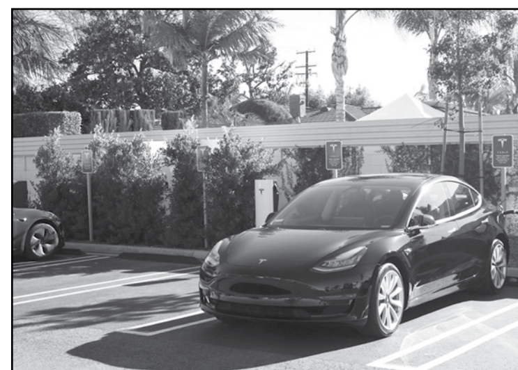
A Tesla charging station at Lakewood Boulevard and Gallatin Road. Photo by Alex Dominguez
