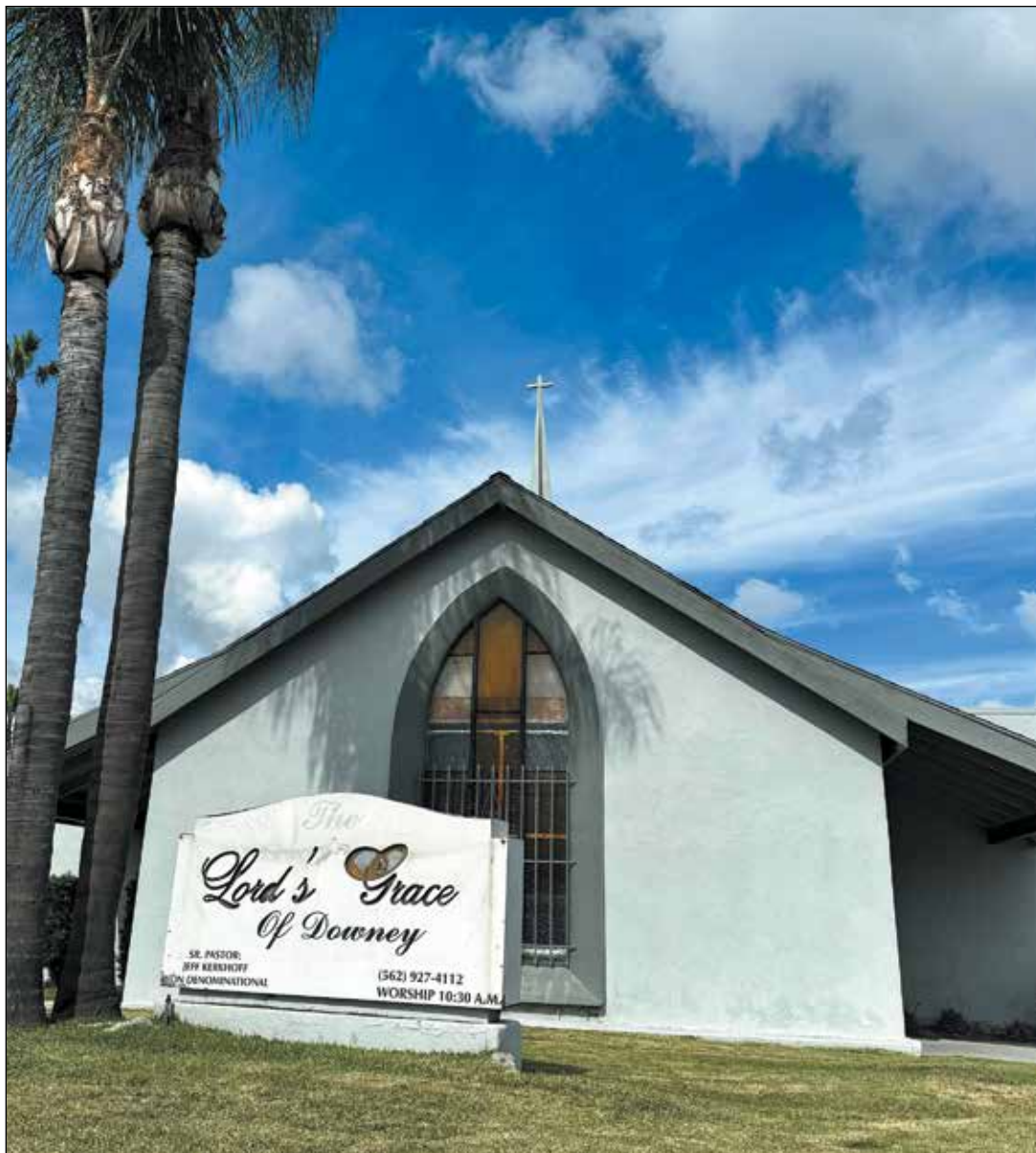
The Downey Planning Commission is expected to consider a developer's proposal to redevelop Lord's Grace Church with 33 townhomes. Photo by Eric Pierce
